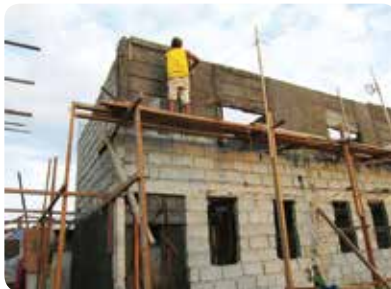
Gawad Kalinga Development Foundation, Inc. の支援で進む住宅建設
